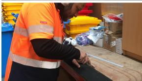
SpillTech® Economy Bunding comes in 2 meter lengths. Before applying the adhesive cut the bunding to the desired length ensuring a tight fit from wall to wall so there are no gaps for liquids to pass through. SpillTech® Economy Bunding can be mitred to create corners if desired
