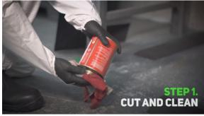
Make sure the surface you wish to adhere the SpillTech® Economy Bunding to is clean and dry before using the adhesive.
